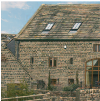
Stone slate, EDW flashing.
