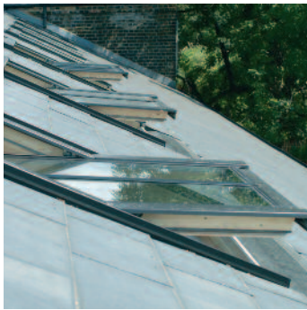
Slate roof, EDN recessed flashing.
