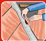
Adhering tiles or tile pieces to valleys
