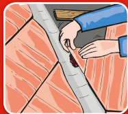
Adhering tiles or tile pieces to valleys
