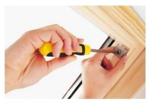
I. Left and right blind mounting plates are screwed into place.
