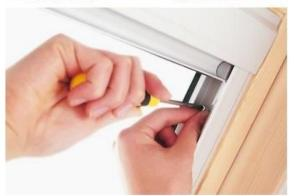
3. Finally, the two aluminium blind guides are slotted into the blind unit and screwed to the frame. It's as simple as that!
