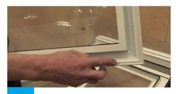
When fitting the roof vent sash position the sash into place with the integrated hinge channel.
