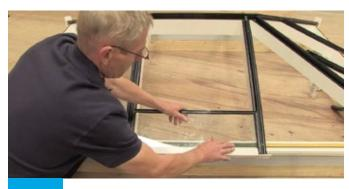
Fix glazing end cover and locate glazing behind rafter end stops.
