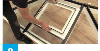
Place the female muntin bar under the glass unit and press down.
