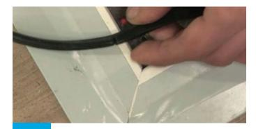
Snip the wedge gasket internally at the corners.
