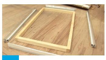
Check that the kerb is square by measuring equal distances from corner to corner. Layout the ringbeams to the correct side of the kerb.
