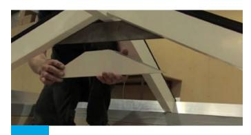
Fix the gusset cover over the hidden tie bar. Secure with screw.
