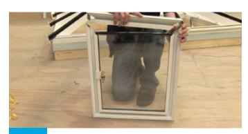
Locate the side of roof vent sash by slotting the corner cleats into the adjoining internal chambers.
