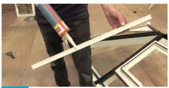
Seal both sides of the external male muntin bar close to the edge and press into position. On wider roof vents have someone push from the inside to prevent deflection.
