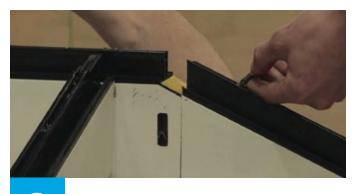
Tighten pre-fixed screw to secure the bell rafter.
