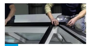
Centralise the ridge pressure plate between the rafter pressure plates.
