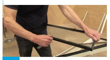
When fitting roof vents always remove foiled or plastic tape from surface of units before sealing.
