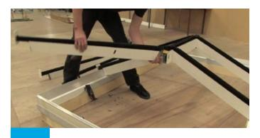
Loosen off the top hip bracket screw and position into the slot provided.
