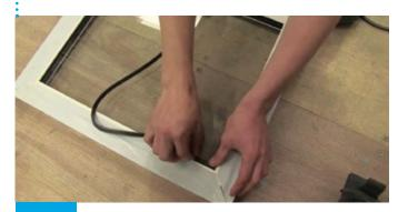
Take the wedge gasket and starting at the corner push it in between the glazing and aluminium vent.
