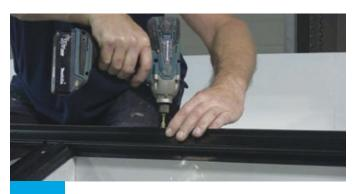
Fix the ridge pressure plate centrally to the main ridge body with screws.
