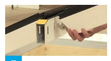
Where there is no hidden tie bar position the bracket into the slot on the ridge and fix rafter with screw.
