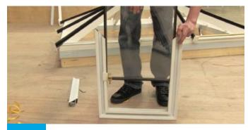
Slide glazing into roof vent sash and press down.
