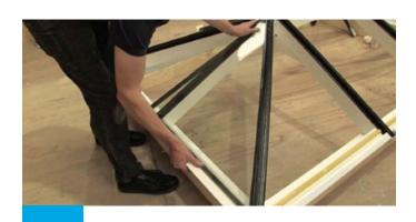
Lift glass into place behind the rafter end stops and press down glazing.
