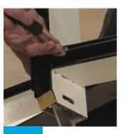
Screw down the top screw to secure the rafter bracket. Place the rafter bracket into the slot on the ridge opposite.
