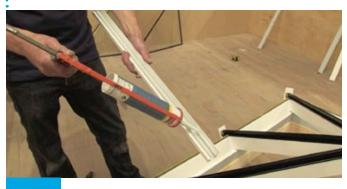
Run a bead of sealant along the top leg of the glazing end closer. Always use the correct sealant.
