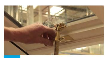
Locate the spindle and tighten bolts to secure.
