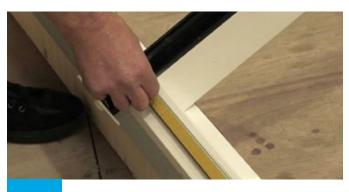
Remove cover tape from double sided tape on the glazing shelf.
