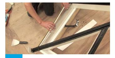
Once rafters are fixed, remove the foam boards and locate the glazing shelf.
