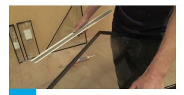
Glue packers into the bottom of the glazing end closer. Slide glazing end closer over the bottom of the glazing.
