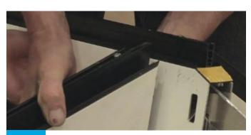
Locate into position with the top rafter bracket and tighten the screw.
