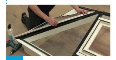
Locate the hip pressure plate centrally over the hip rafter and fix down with screws.
