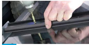
Position the central pressure plate over rafters. Screw the pressure plates through the predrilled holes provided.
