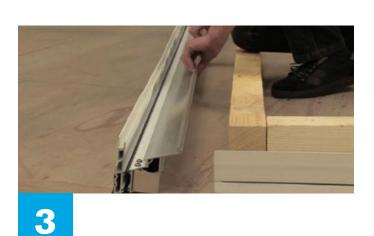
Remove the ringbeam flaps from the ringbeam.
