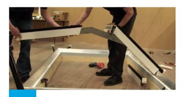
Slide the adjacent rafter over the steel angled bracket.
